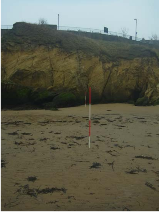
Plate 3 – Survey photograph 1aNTDC05_20140403_Up3.JPG
